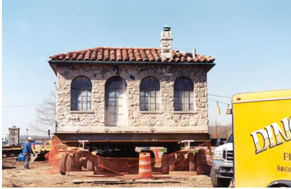
Movers relocate the 1931 Wright Field guard house to the new Gate 1B location
