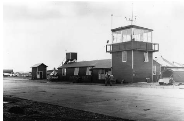
Patterson Field control tower, 1940
