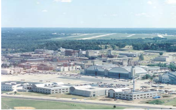
General James H. Doolittle Acquisition Management Complex dedicated in 1994
