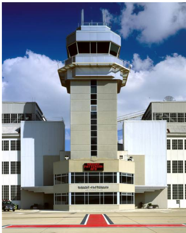
Wright-Patterson's new control tower, 2003
