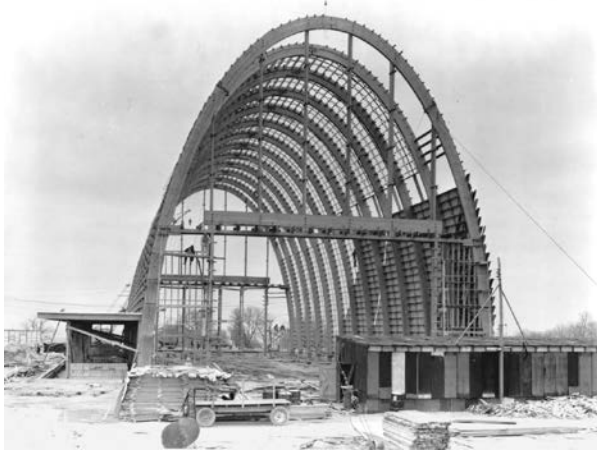
When completed, the all-wooden Radar Test Facility (Building 821) supported pioneering stealth technology research
